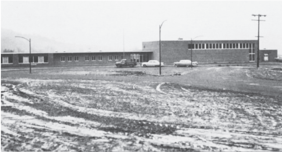
The school as it nears completion, 1958-1959
